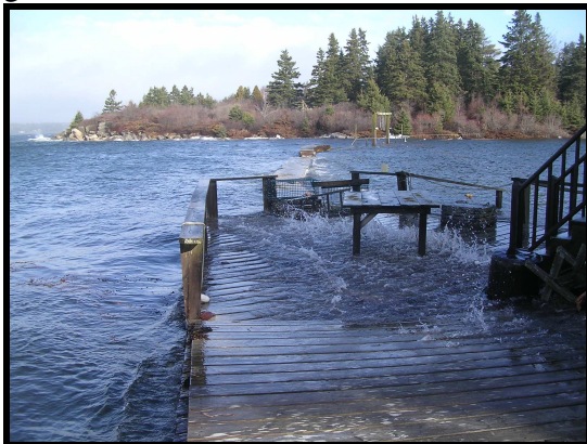
High tide at Friendship Long Island Lobster Pound on December 3, 2009 – one of the days the tide didn't fall low enough to sample juvenile lobsters. The dam is underwater (see 1900's pound photo above for comparison with how things should look), the wharf in front of the house is being rocked up and done and taking the front porch stairs for a ride.
